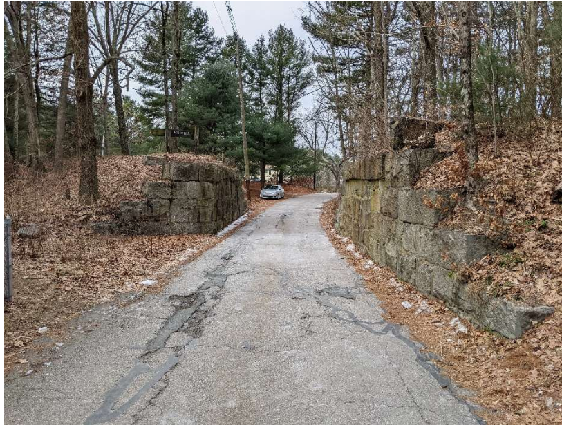
Hill Street facing west. Note stone structures on both sides of road at corridor crossing. The abutments from the former railroad bridge are listed on the MHC inventory of historic structures.
