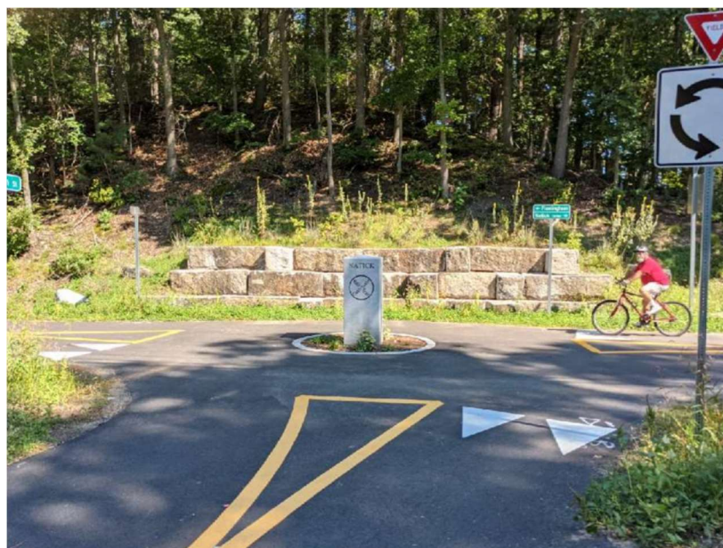
Example of the reuse of stone blocks for slope stabilization and seating on the Cochituate Rail Trail
